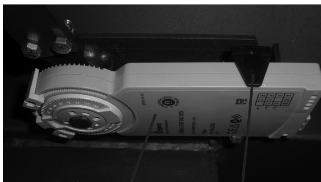
Servo motor Motor retaining clip
