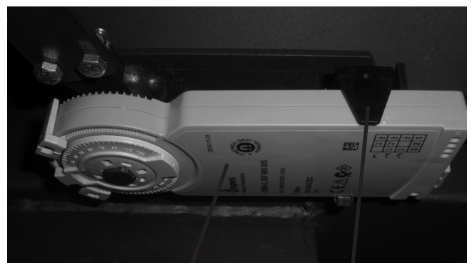
Servo motor Motor retaining clip
