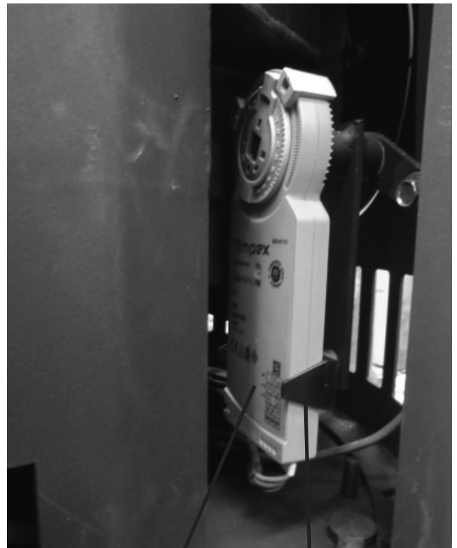
Servo motor Motor retaining clip
